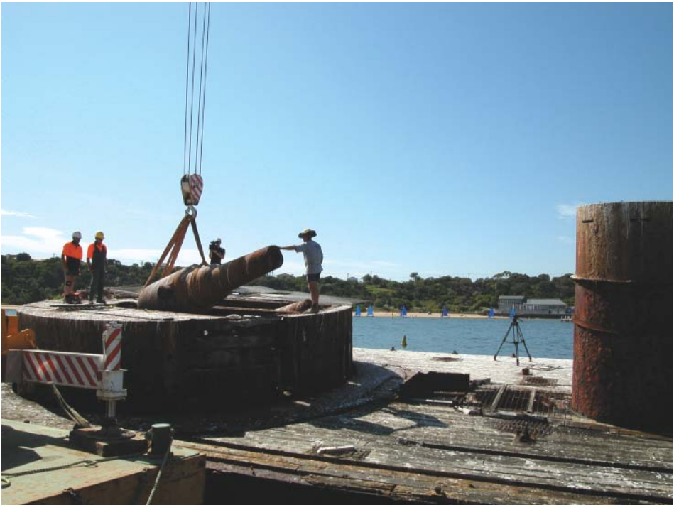
FIGURE 10 Removal of a 16 tonne gun barrel from the aft turret, January 2005, for placement on the seabed.
